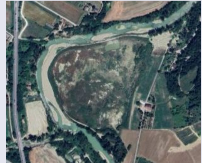
In 2023, after the flood
